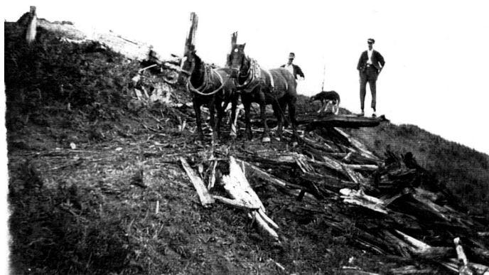
Clearing a blue-gum which fell across Earls Rd beside 'View Point', 1938
