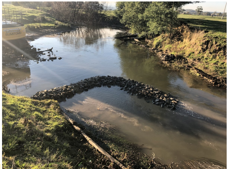
The temporary coffer dam taking shape during the construction phase
